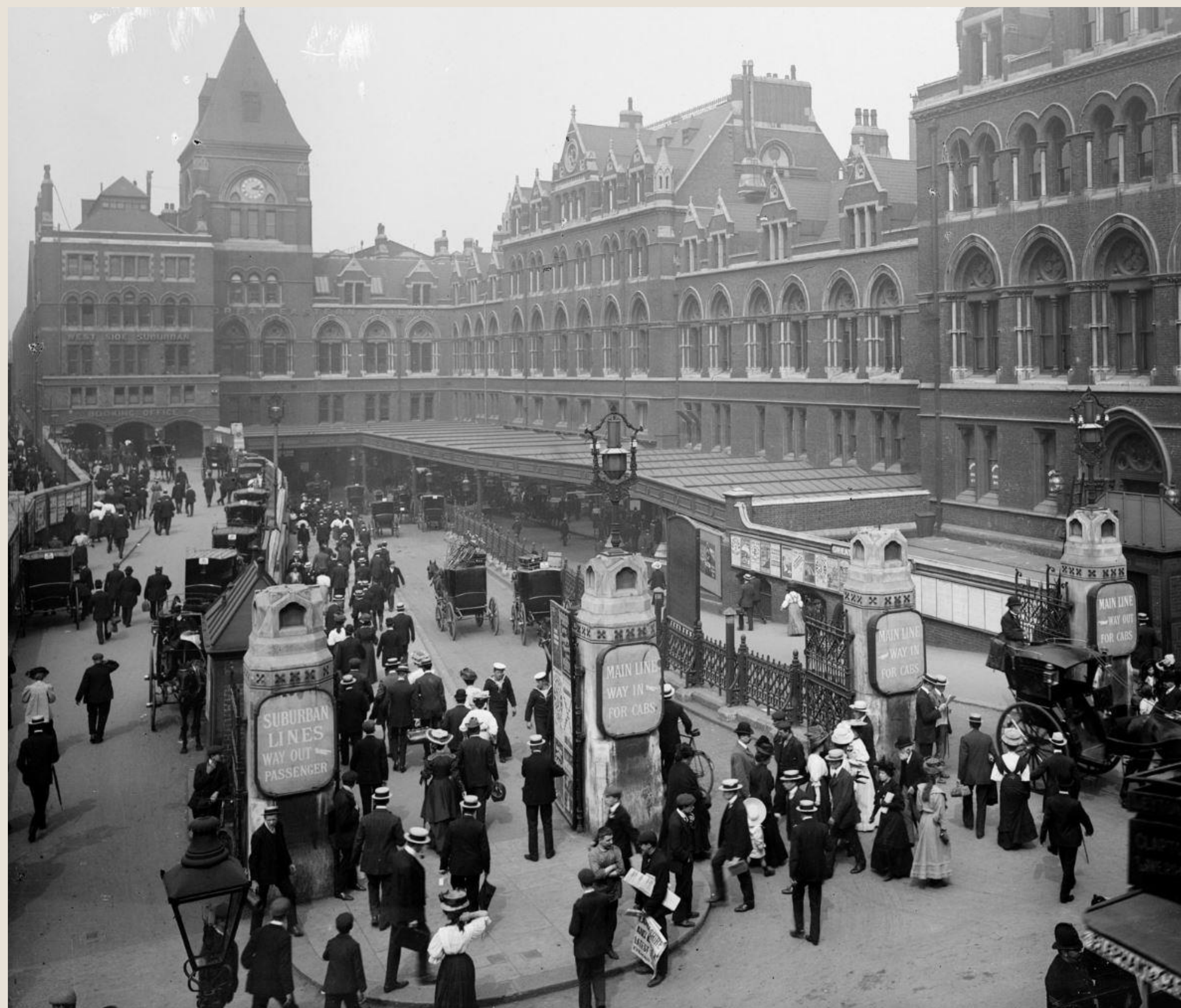
The original station entrance with ramps down to the platform level
