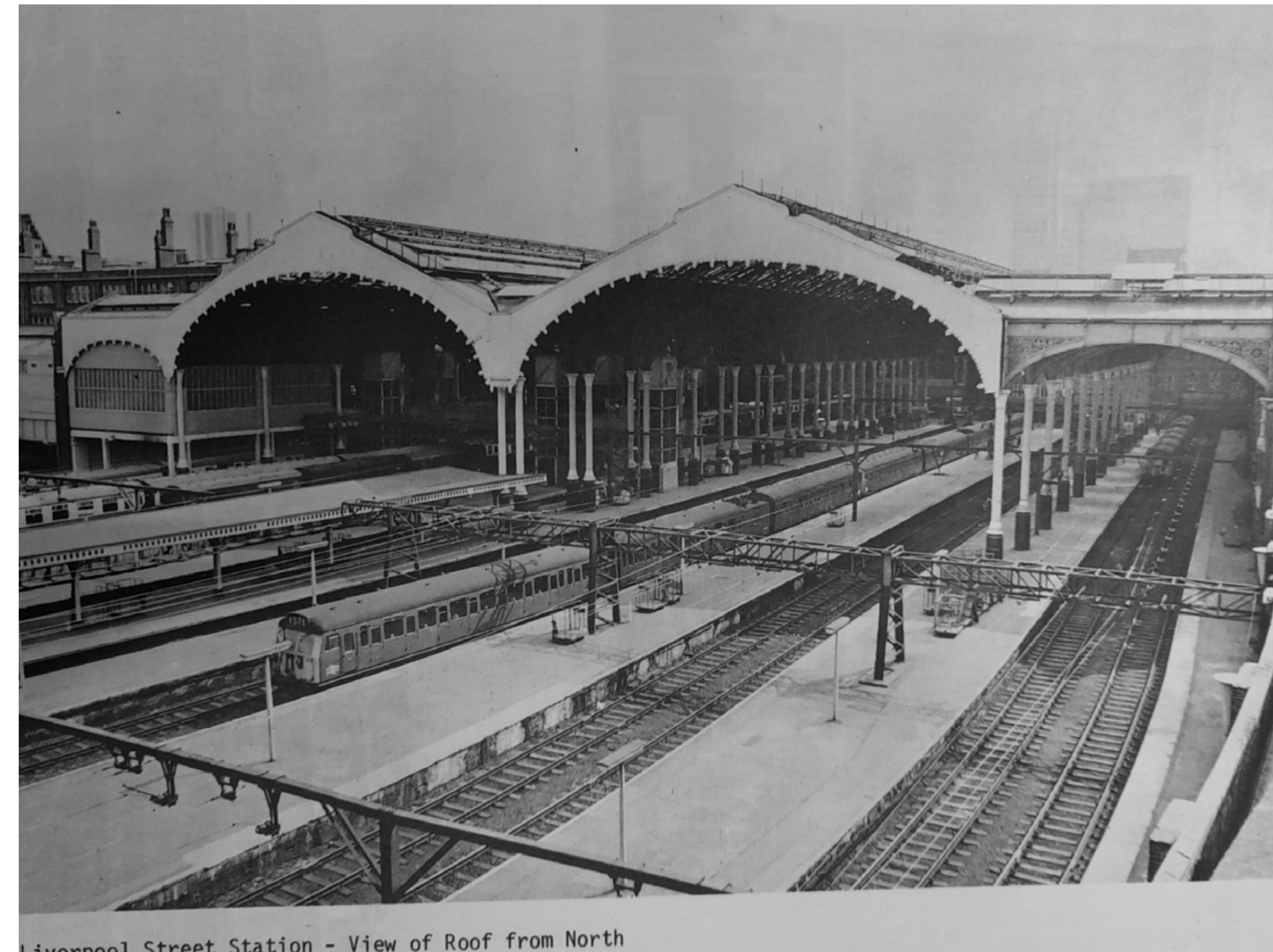
Liverpool Street Station - View of Roof from North
